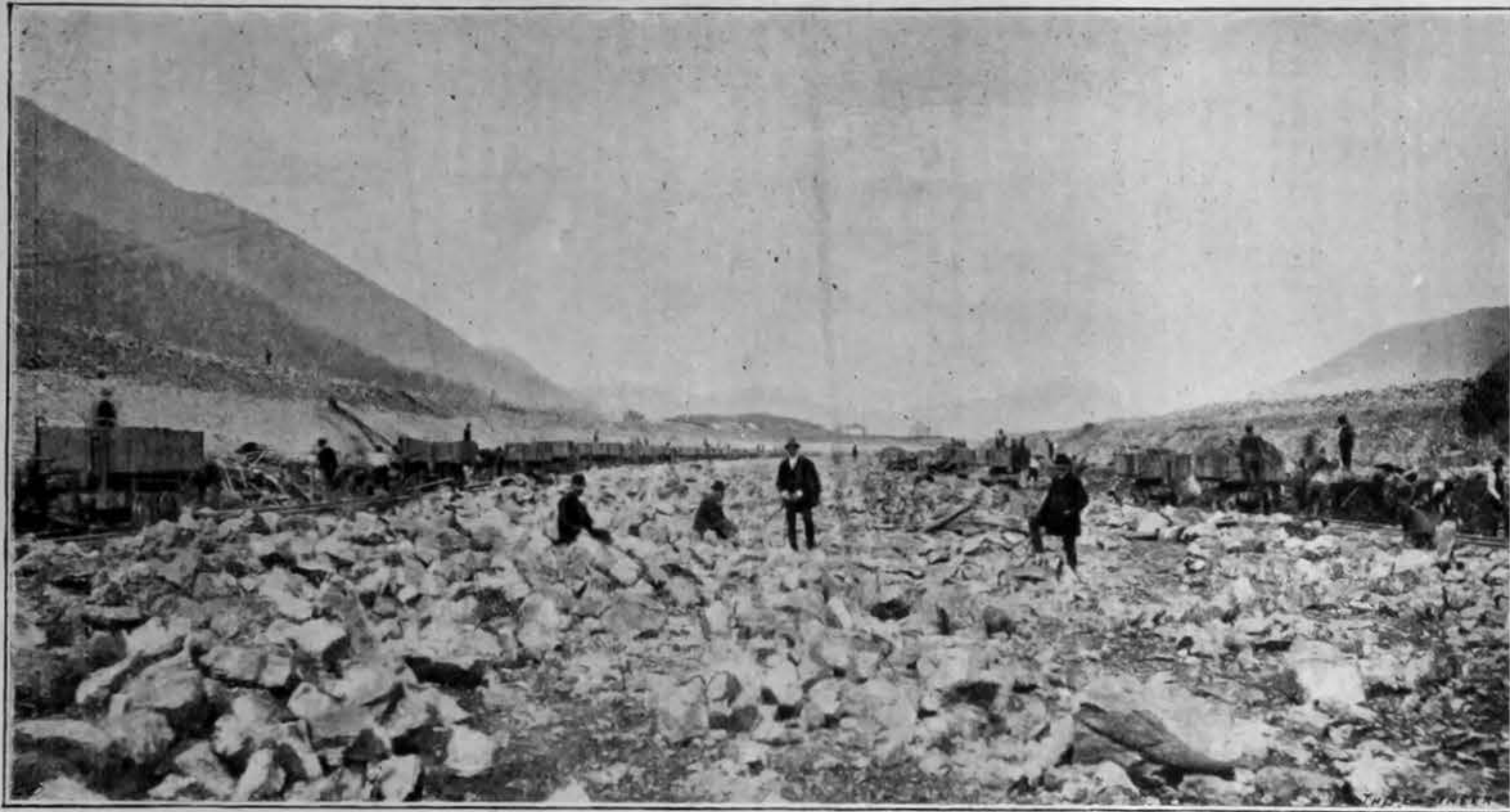
EXCAVATION OF THE CANAL THROUGH THE ROCKS OF THE IRON GATES
